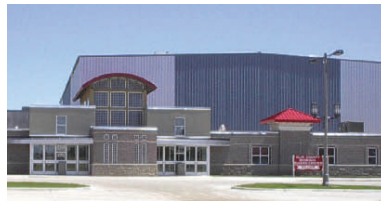
Clay County Regional Events Center
